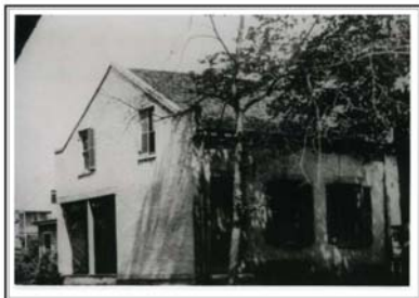
Burch House, Reconstruction
