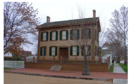
Existing Lincoln House
