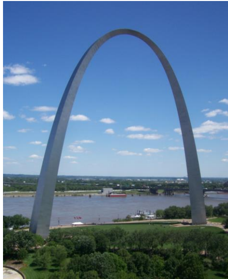
Figure 8, View of the St. Louis Arch and the Jefferson National Expansion Memorial
